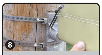
Slide the banner over the poles and use the zip ties through the retainer rings and grommets to secure the banner in place. Adjust the bottom bracket to ensure that the banner is taut.
