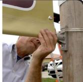
Set the bottom bracket (with the arrow pointing down) to the desired height on the pole. Secure the bracket in place with two release bands.
