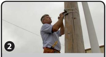
Set the top bracket (with the arrow pointing up) to the desired height on the pole. Secure the bracket in place with two release bands.
