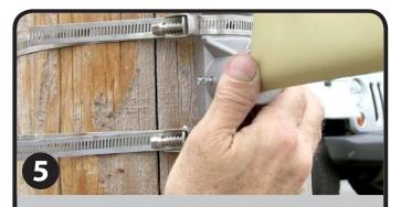
Insert the clevis pins through the open hole.
